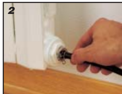
2 Screw on the drain tube provided
